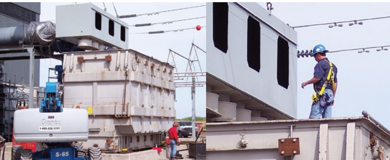
800 MVA Emergency GSU Change Out
