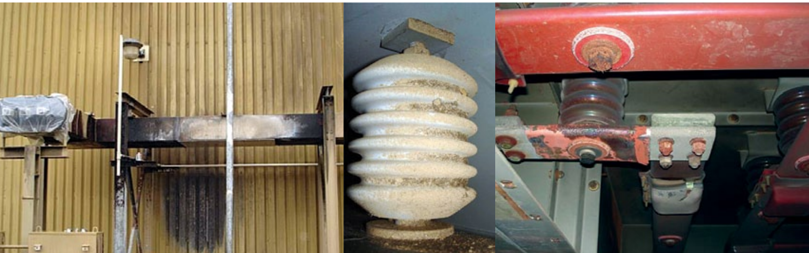
Actual "As Found" site conditions by Crown's Service Personnel
