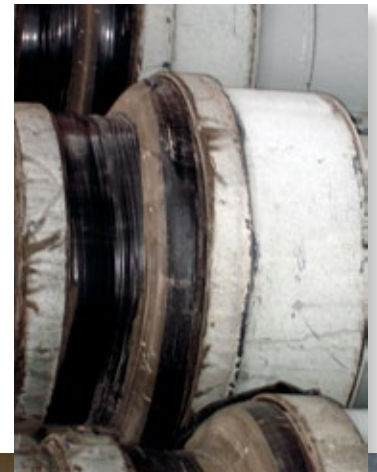
Electricians tape protecting cracked vibration joints
