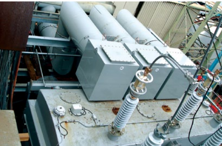
New "throats" now provide bushing access
