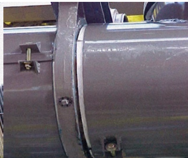
Insulating paper isolates one side of IPB Enclosure
