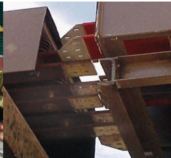
Crown's unique expertise in lining with existing bus
