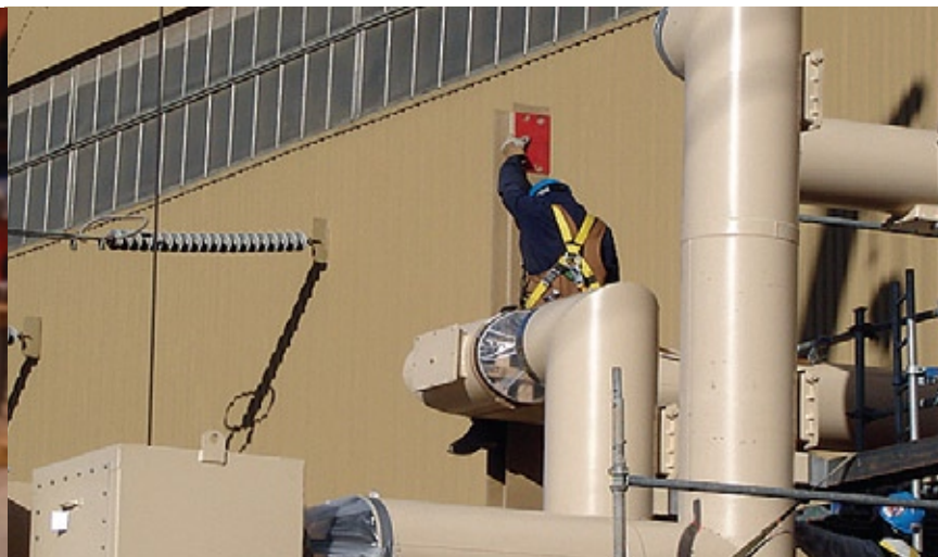
Installation of a new Continuous IPB
