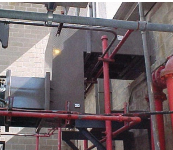
Custom retrofit and upgrade of Phase Seg bus
