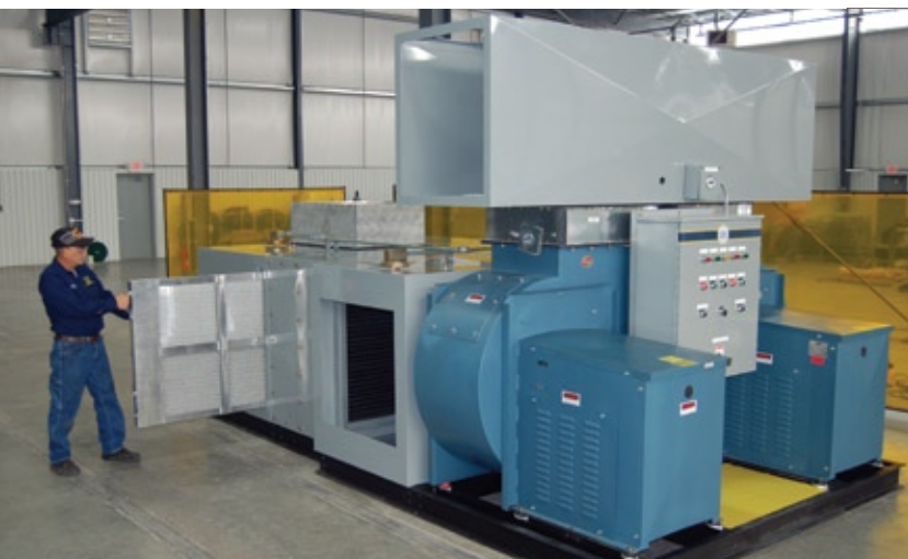
100% redundant 12,000 CFM cooler
