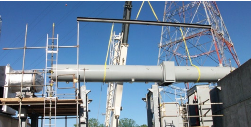
Delivery & pick of a single 50 foot Circular Non-Seg section
