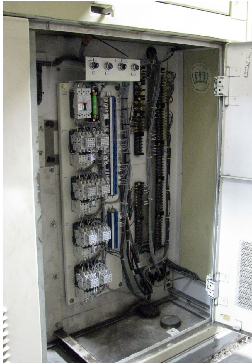
New custom control panel designed for ease of retrofit & wire drops
