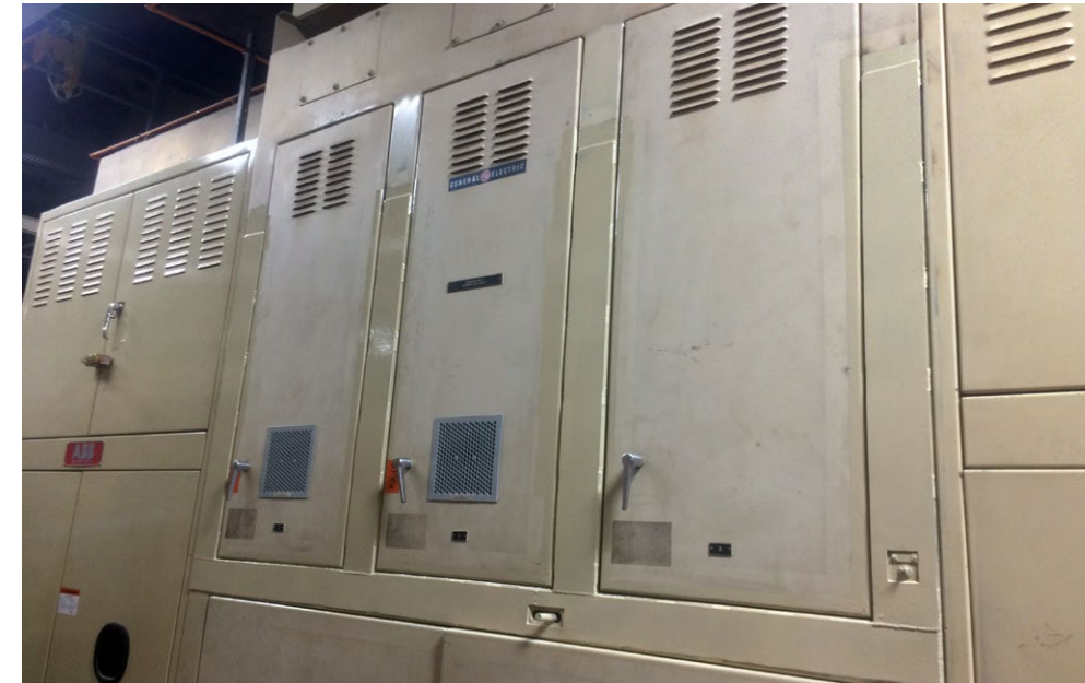
Extremely tight access available for retrofill work
